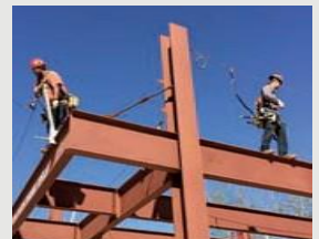
Structure features cantilevered members for stability training.
