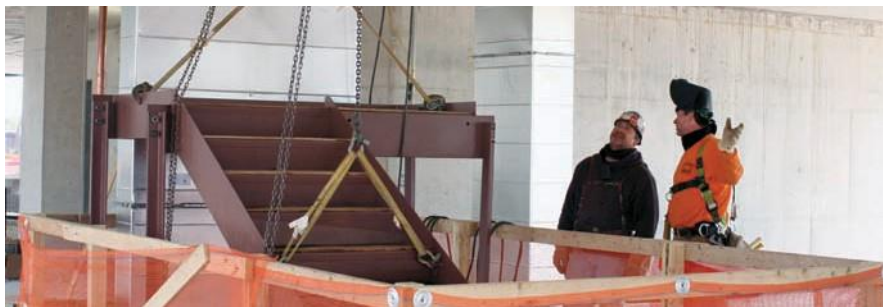
McGregor Top Tread Stair being installed at the One Riverside project in Philadelphia by James McGovern, Local 489 (Scranton, Penn.) and Ken M. Stagemyer, Local 401 (Philadelphia).
