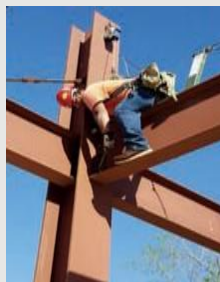
Retractable lanyard anchored to column lug.
